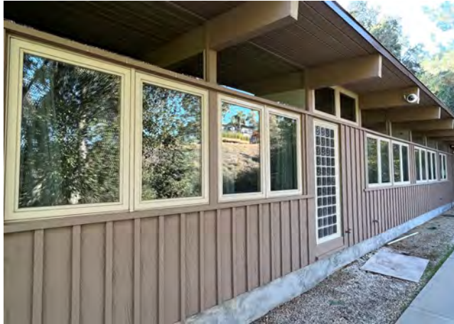
West façade, Baker Residence, facing southeast.
