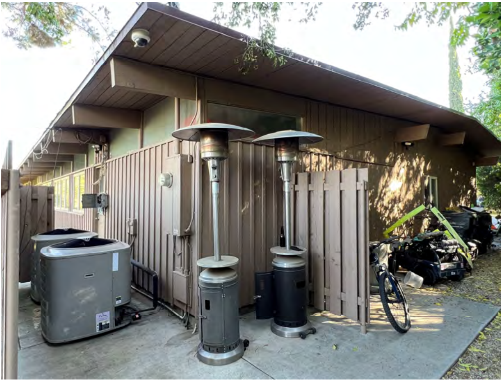
West and East Façades, Baker Residence, facing northwest.
