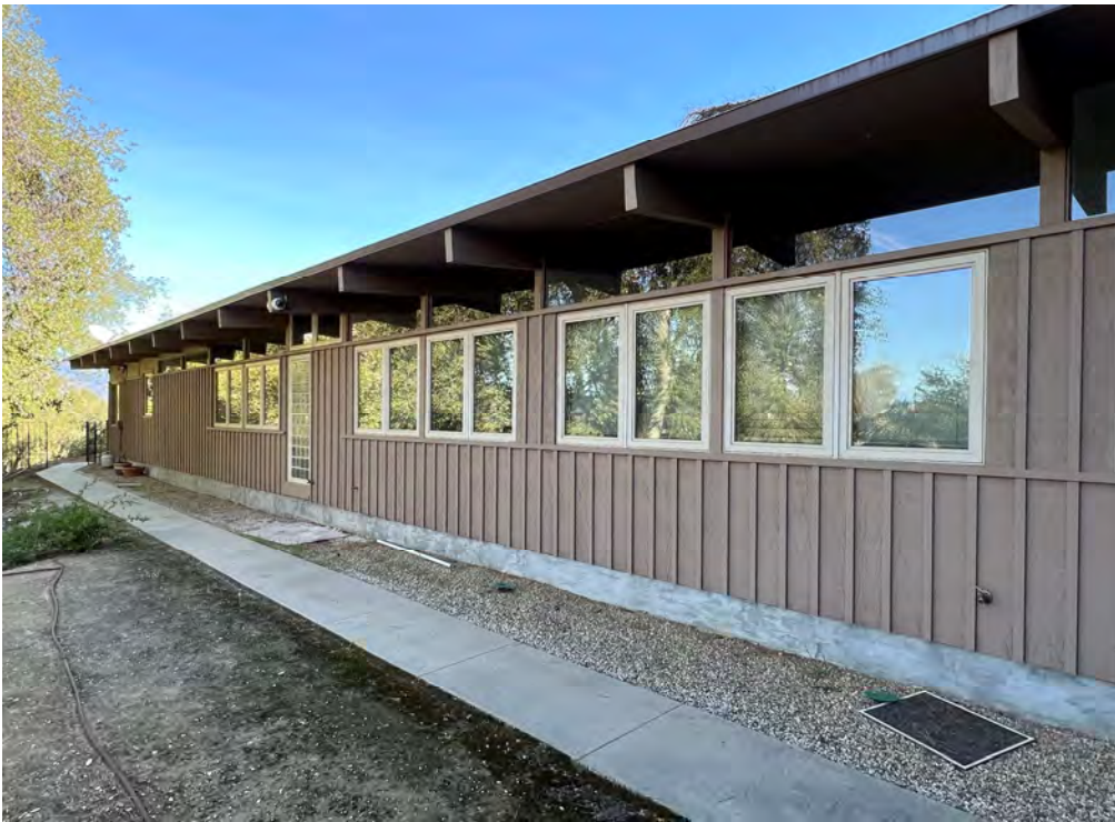
West Façade, Baker Residence, facing northeast.
