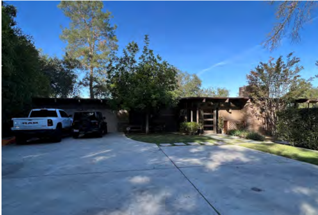
Overview of Baker Residence, East façade, facing west.
