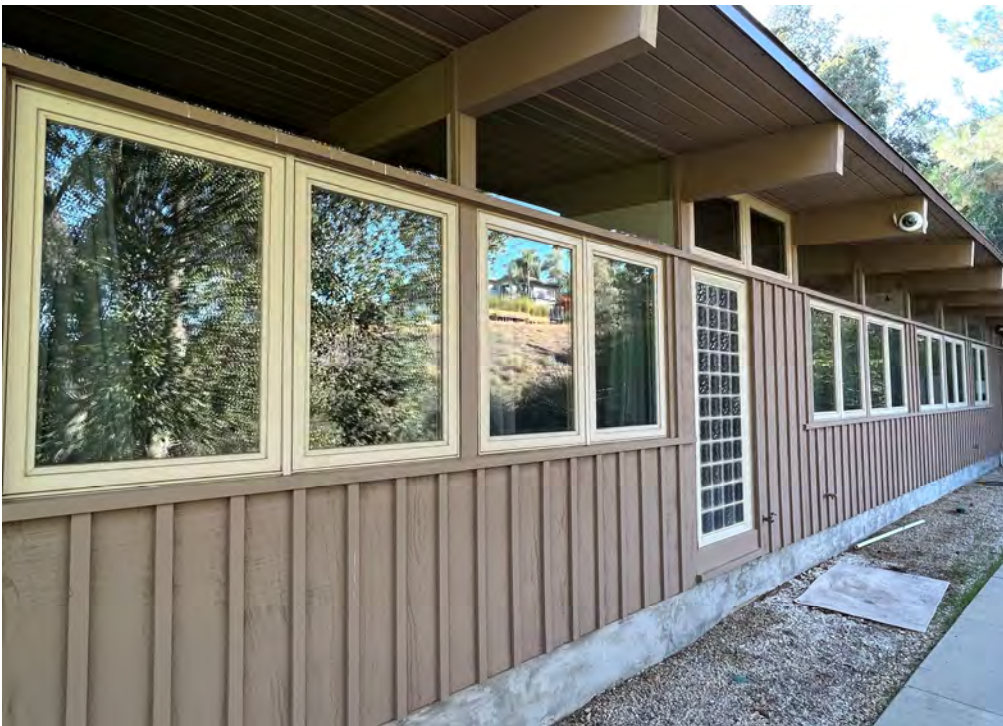
West façade, Baker Residence, facing southeast.
