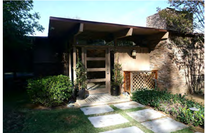
Primary entrance, east façade, Baker Residence, facing west.
