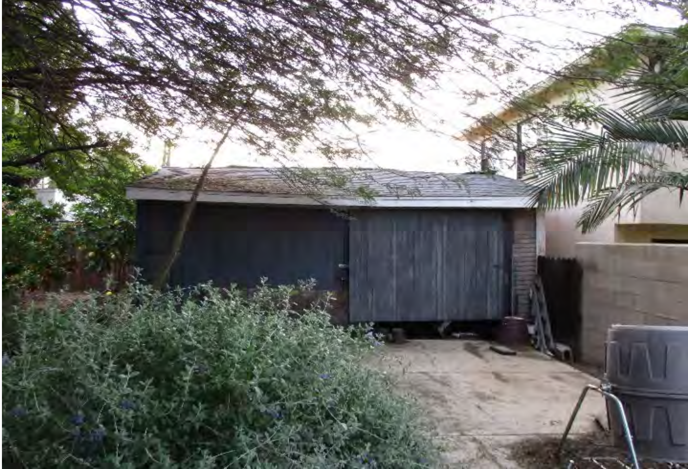
Front (North) Elevation of Garage
