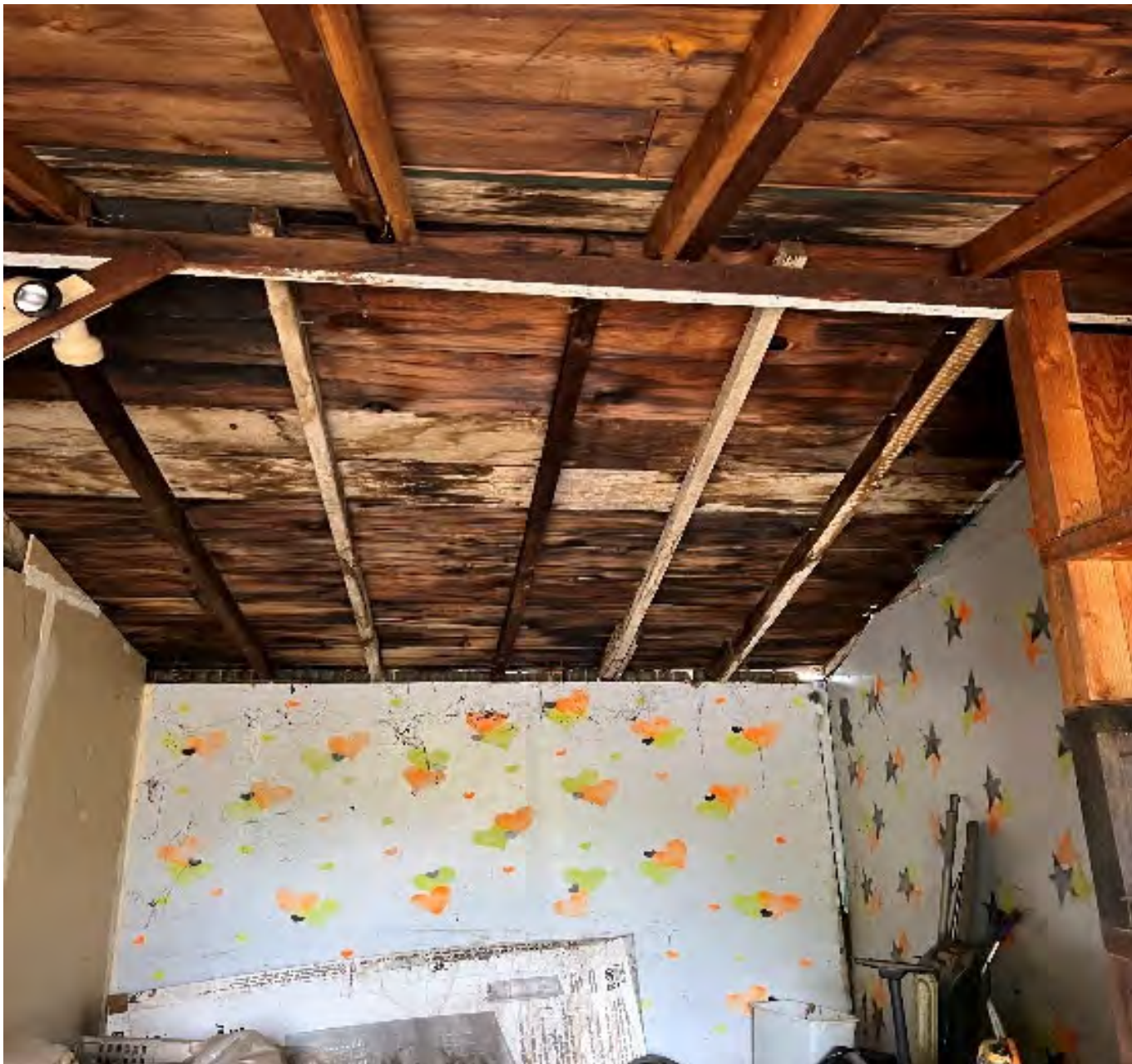
Alternate view of interior roof structure
