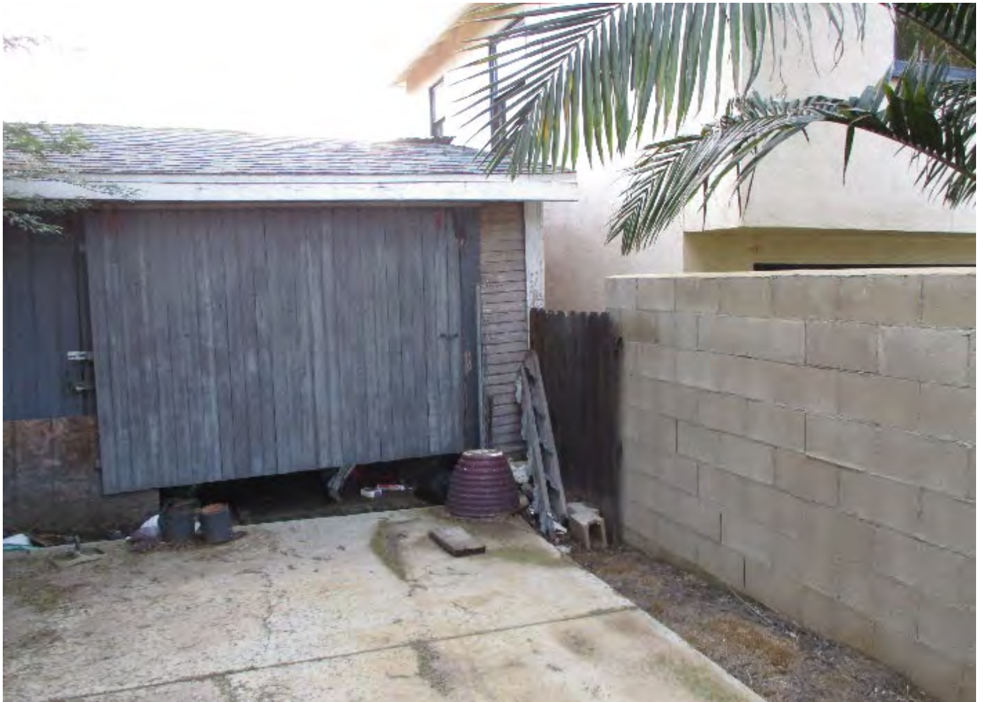
Alternate view of Front (North) Elevation of Garage
