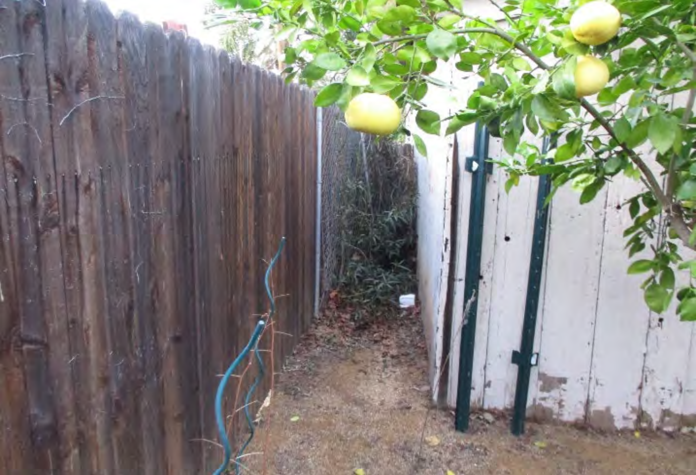
Rear (South) Elevation of Garage at fence
