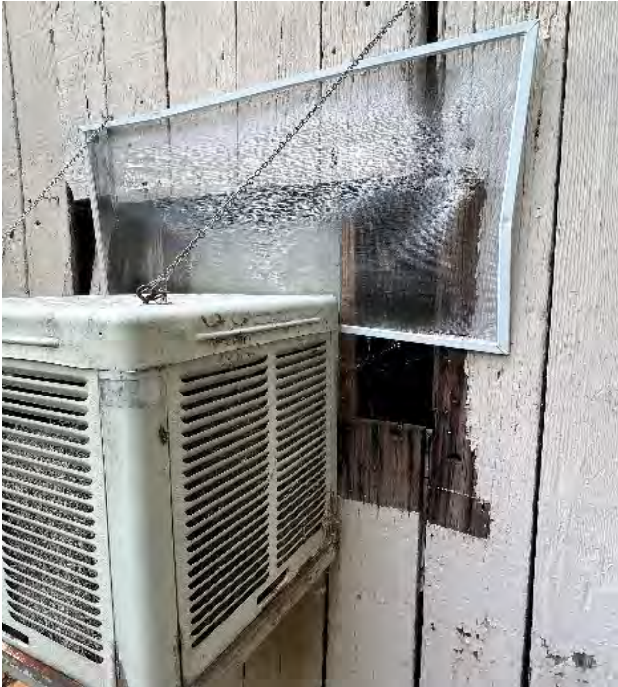
Partial View of east (side) wall at A/C unit
