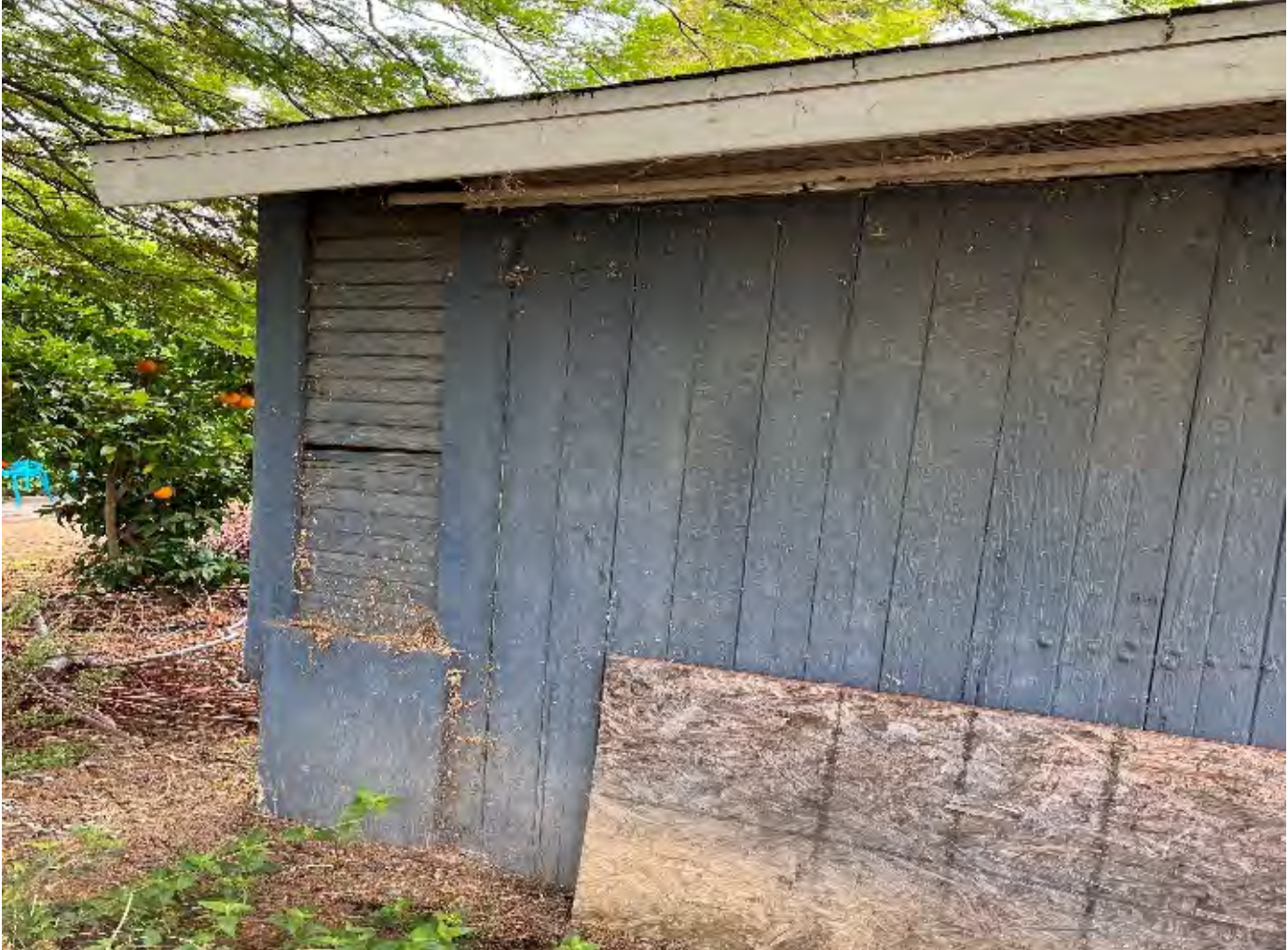
Alternate view of front(north) at east side
