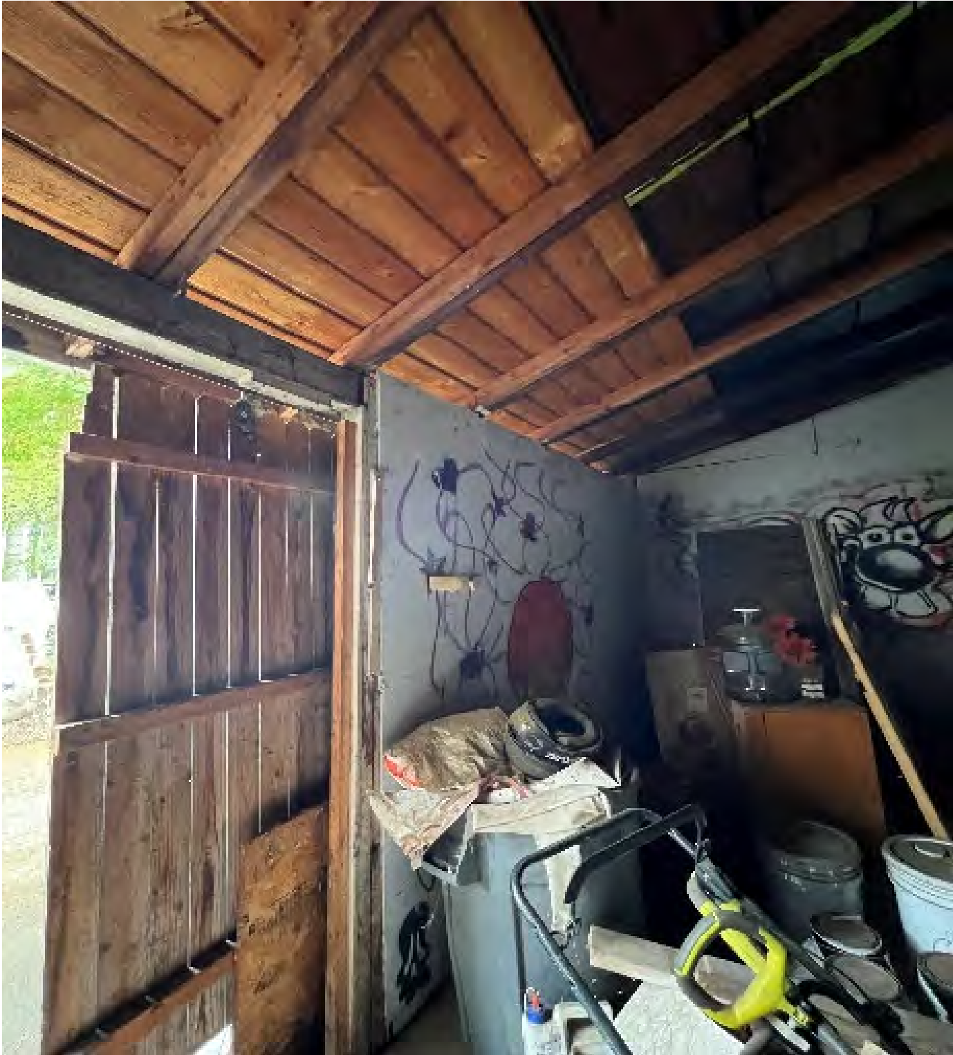
Alternate Interior view of roof structure at garage door
