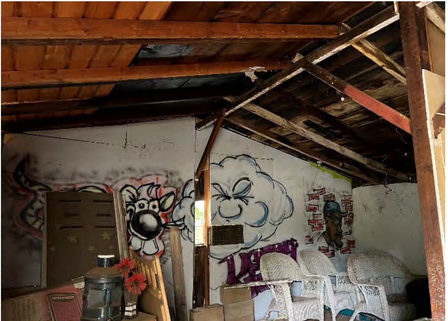
Interior view of interior wall facing south
