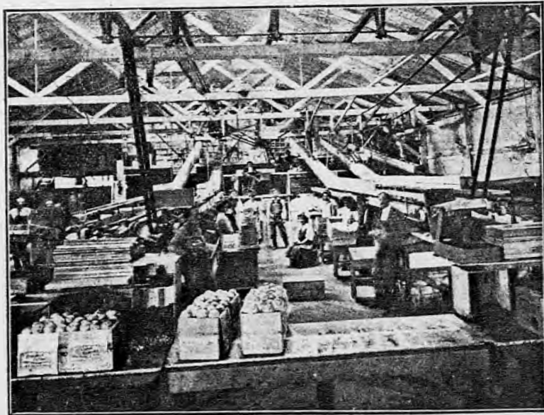
Interior West American Fruit Company's House.
