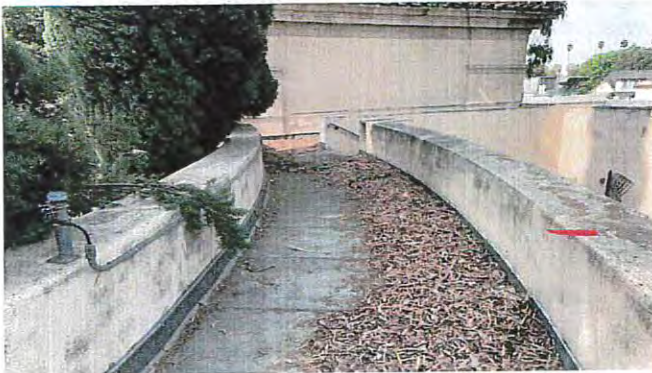
It is recommended to encapsulate the entire section from the outside edge of the parapet wall to the opposite outside edge after prepping the top of the parapet wall and applying a self-adhering divorcement sheet.
