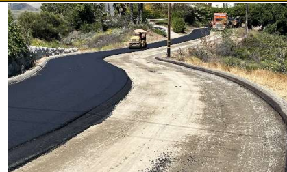
Paving on cement treated base on Edgemont Dr.
