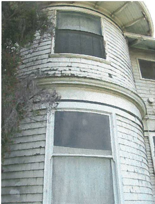
Closeup of curved windows on tower.
