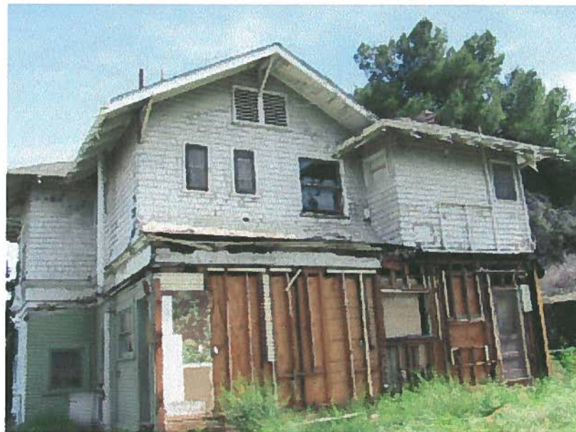
South-facing rear of house
