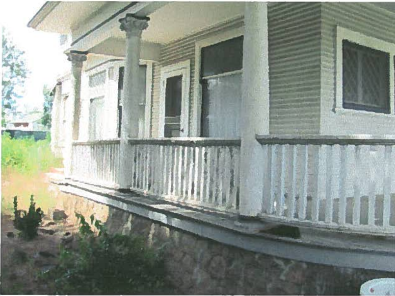
East side; original rock foundation
