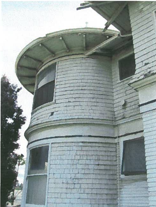
Tower with rafters
