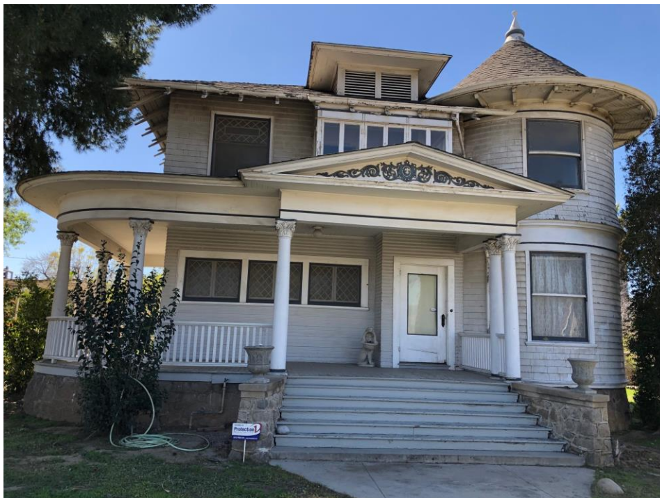
P5a. Front (North) View
